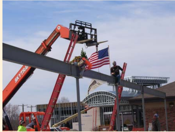
Final I-Beam finds it's home!
